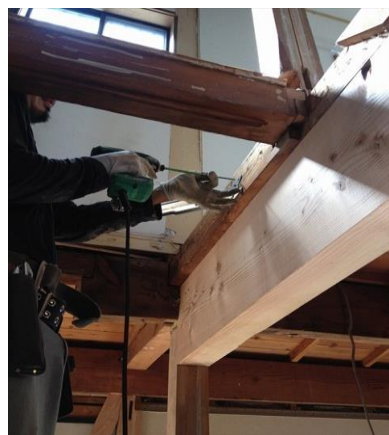
まくら梁補強
