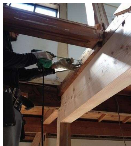
まくら梁補強
